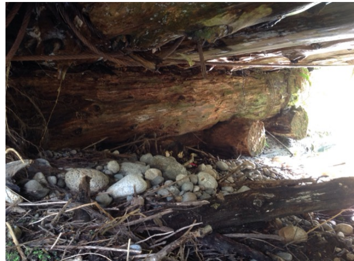
Left Bank Abutment when facing downstream
