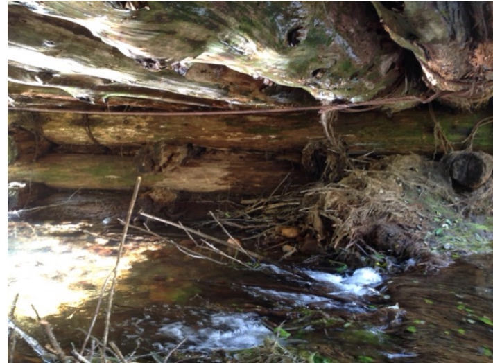
Right Bank Abutment when facing downstream
